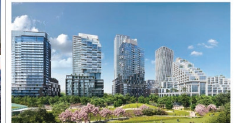
A revamped park, a new community centre, and 8 new towers make up the massive redevelopment at Dufferin and Dupont streets. (ELAD Canada)
